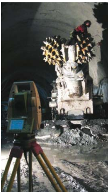
The Roadheader system in use with a Leica TPS1200 Total Station
